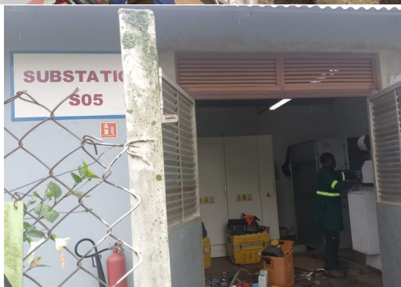
FIGURE 1 I LONG TEAM GETTING ACCESS TO SUBSTATION NO.4 AND NO.5
